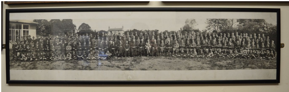
Lincoln School during the Great War on the Sewell Road site now the hospital car park The house in the distance is still there surrounded by nurses' homes Photograph by Catherine Forbes
