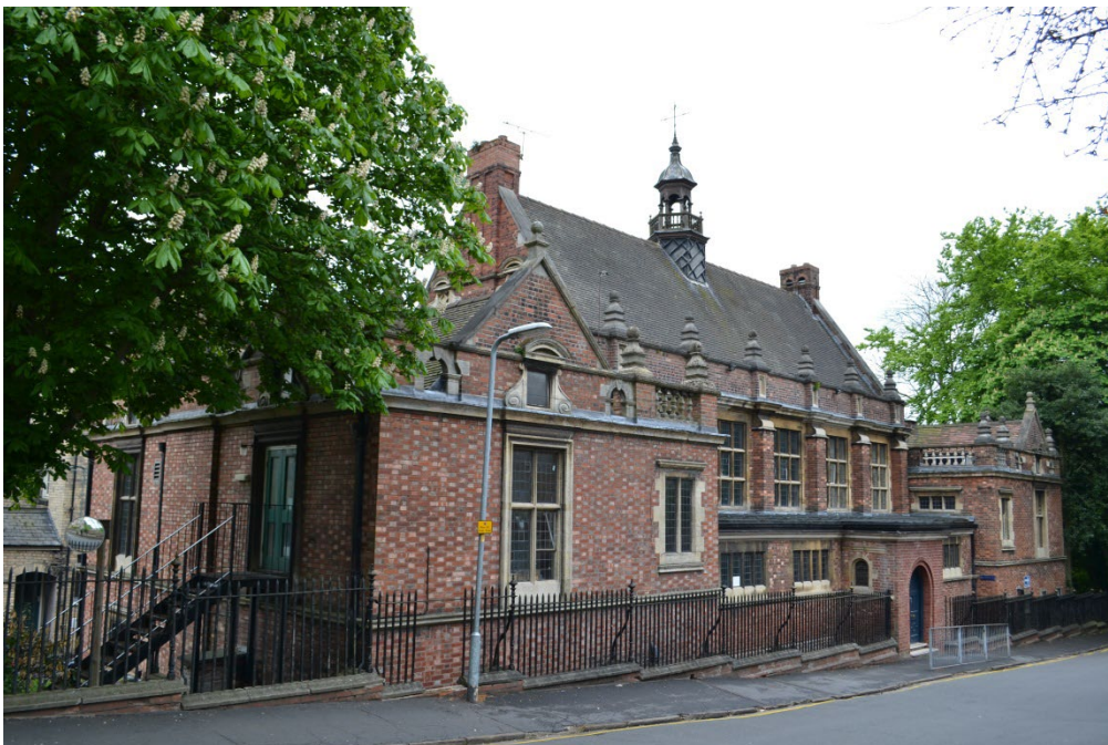
Former Lincoln Grammar School building on Upper Lindum Street, now part of The Minster School
