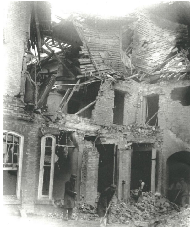
Coldbath House in Ruins Photograph from Lincoln Central Library Collection
