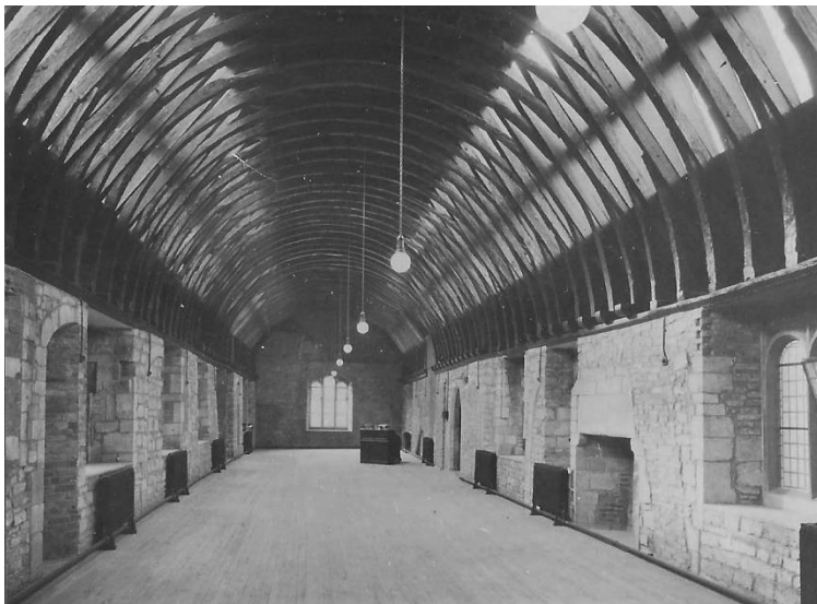
A 20 th Century view of the Greyfriars Schoolroom looking towards Broadgate
