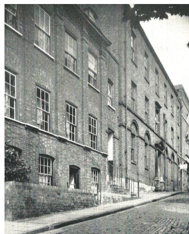
The Bluecoat School on Christ's Hospital Terrace
